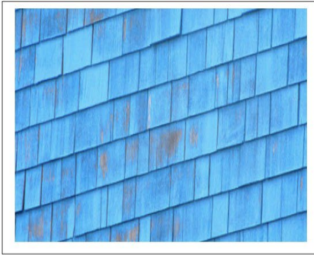
Examples of chipping paint, deterioration, breaks and gaps (leading to further damage) in violation of Code
