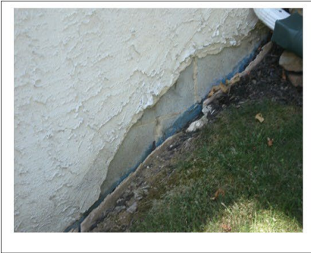
Damaged-Decaying Stucco
