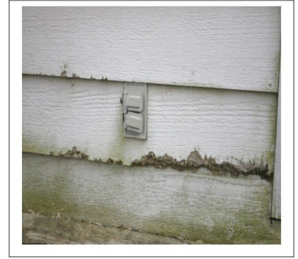
Examples of chipping paint, deterioration, breaks and gaps (leading to further damage) in violation of Code
