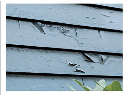
Examples of chipping paint, deterioration, breaks and gaps (leading to further damage) in violation of Code
