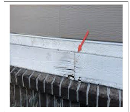
Examples of chipping paint, deterioration, breaks and gaps (leading to further damage) in violation of Code
