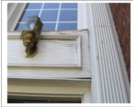
Examples of chipping paint, deterioration, breaks and gaps (leading to further damage) in violation of Code
