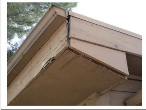
Examples of chipping paint, deterioration, breaks and gaps (leading to further damage) in violation of Code
